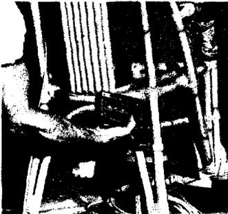
**FURNITURE MAKER CUTS LABOR COSTS 30%** applying 1/4" plastic strips to rattan joints. He changed from brass nails to Bostitch T5 stapling tackers. He gets more secure fastening, too.
