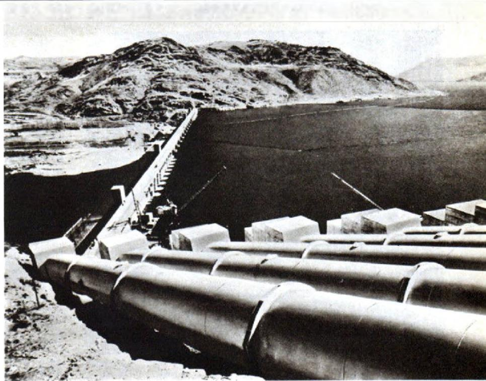
**PART OF THE WORLD'S LARGEST** pumping plant are these huge steel discharge lines for Grand Coulee on the Columbia River in Washington. Each line is 12 feet in diameter, was fabricated by United States Steel. Only steel can do so many jobs so well.
